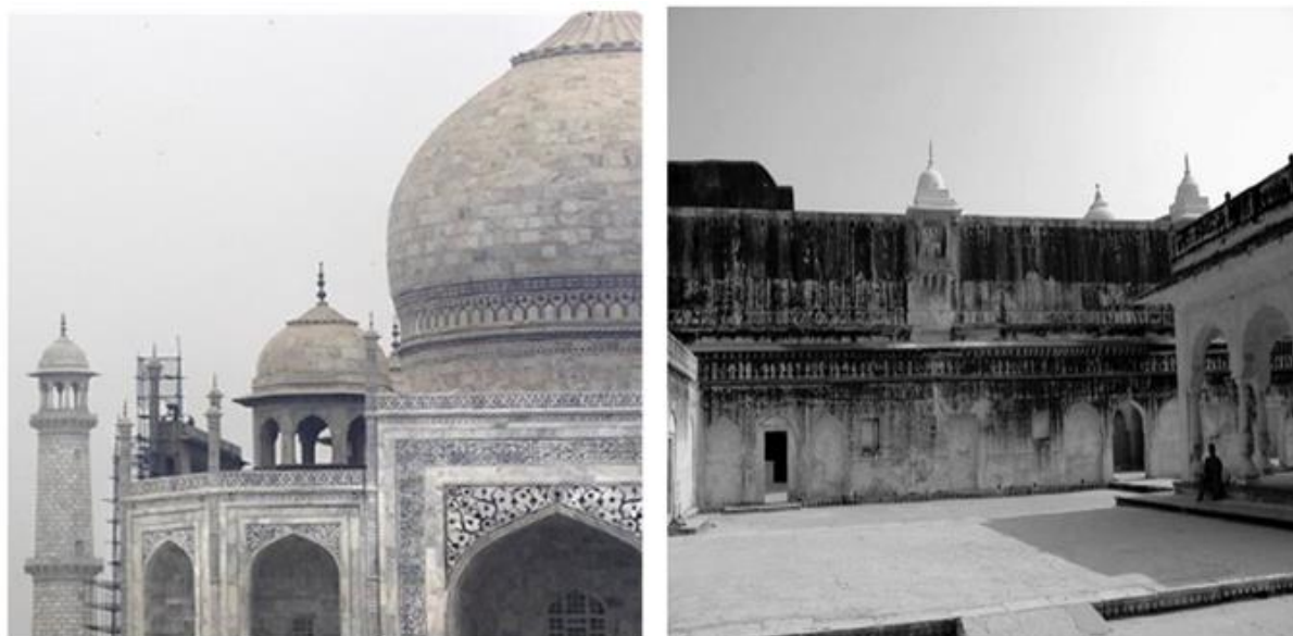
Figure 1. 20: Discolouration on monuments in humid climate (Adapted from (Stephanie Scheerer, 2009) www.washingtontimes.com ).
