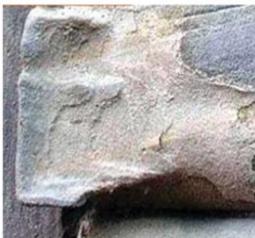
Figure 1. 5: Evidence of flaking on marble building (Adapted from (V.Verges-Belmin, 2008)).
