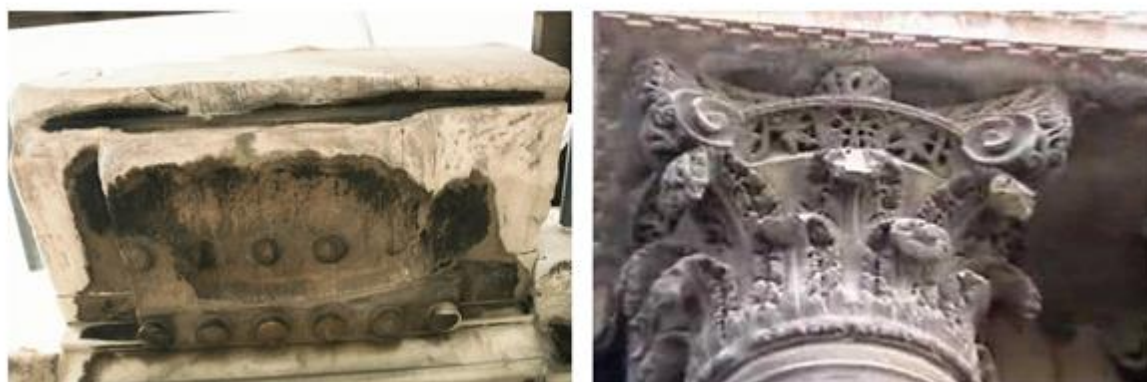
Figure 1. 14: Effects of Sulphation on marble capitals (Adapted from: www.ysma.gr/en/conservation-degradation-phenomena , https://pubs.usgs.gov ).
