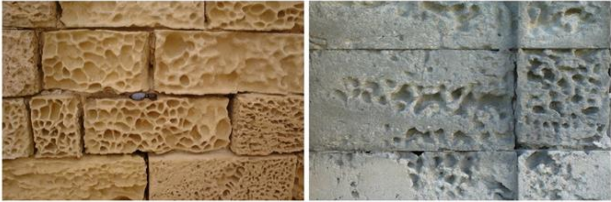
Figure 1.17: Effects of alveolisation on exterior walls of building (Adapted from: www.buildercorp.pl , www.wikipedia.com ).
