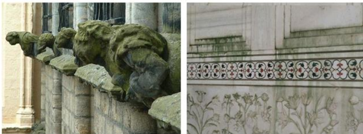
Figure 1. 10: Algae on exterior wall due to water leakage and humidity (Adapted from: http://www4.rgu.ac.uk , http://www.lefigaro.fr ).
