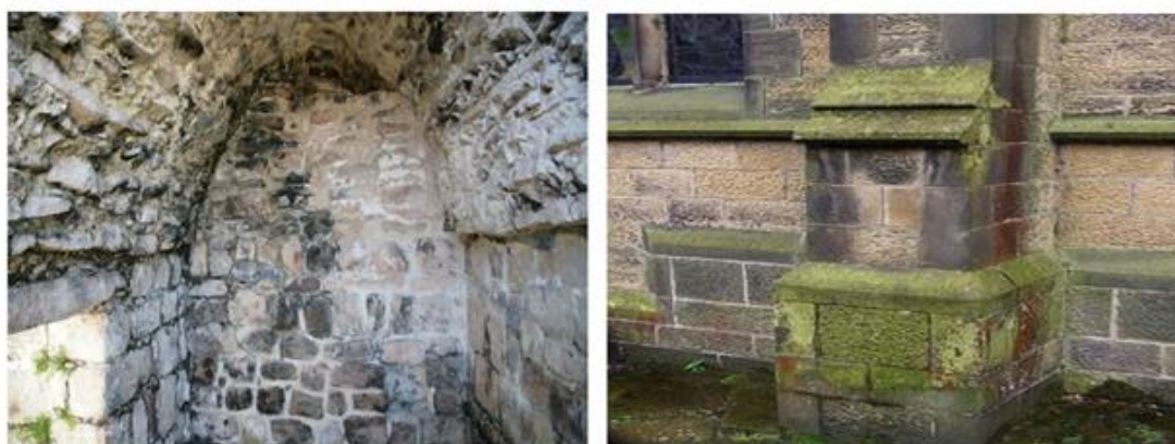
Figure 1. 9: Cyanobacteria on interior and exterior walls (Adapted from: https://bakalchen.wordpress.com , right, https://www.qub.ac.uk ).
