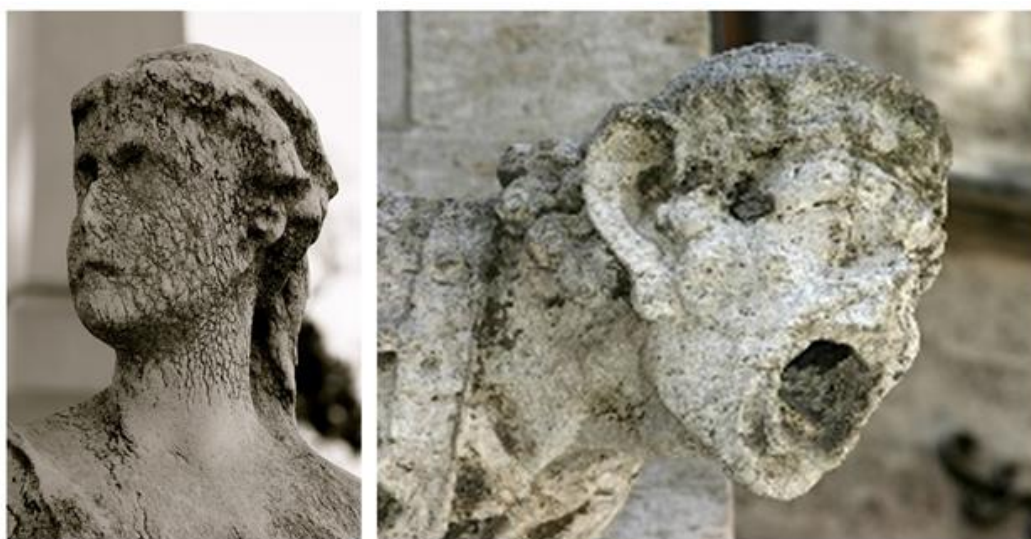
Figure 1. 15: Effects of weathering and erosion on stone (Adapted from www.marsnow.info , www.pinterest.com.mx ).
