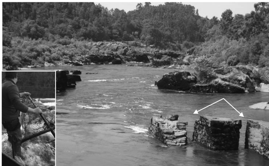
Fig. 4. Fishing weirs (“pesqueiras”) in Lima River. The white arrow shows the slots where the traps are placed (see detail in the left corner) (Photo “pesqueira”: B.Quintella; photo fisherman: G.Cardoso).
