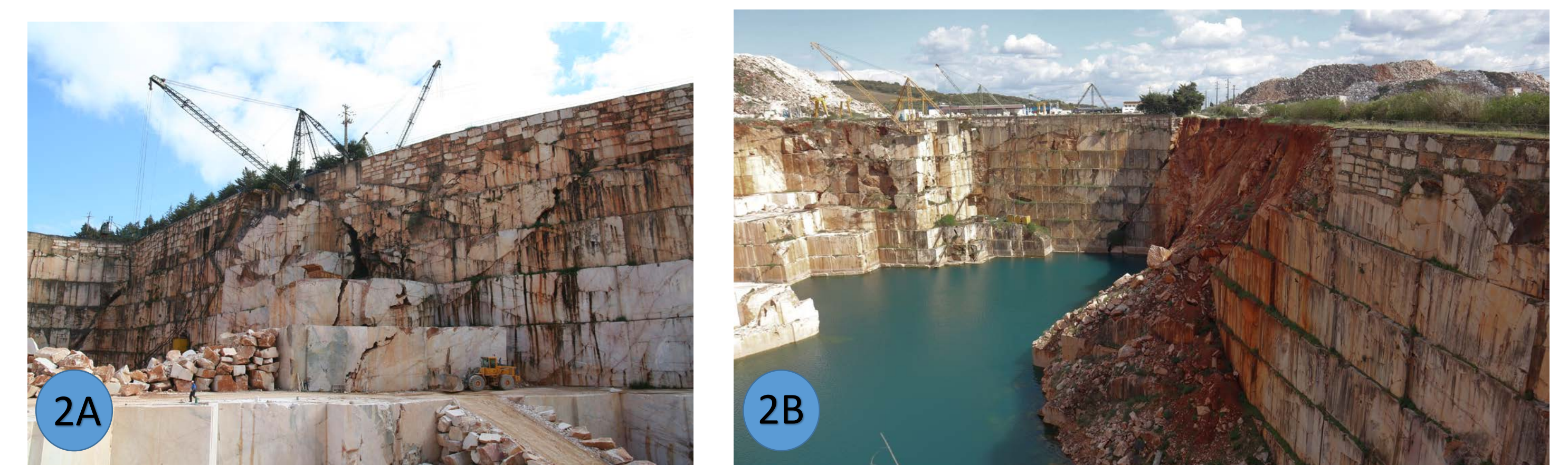
(2A) Quarry located next to the municipal road M255 that would eventually collapse (2B) at 15:45 on November 19, 2018, with an approximate length of 100 m. As a detail, note the lack of arboreal screen on the crest of the slope in (2B).
