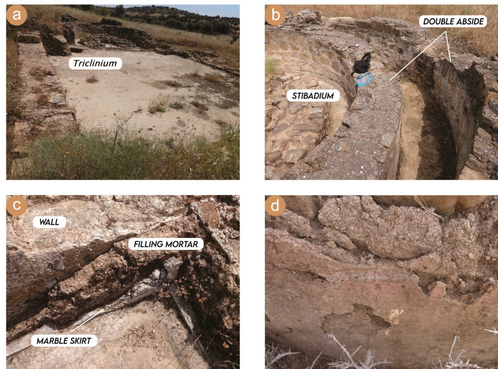
Figure 2. An overview of the different parts of the site: (a) a perspective view of the main banquet hall (i.e., triclinium ); (b) walls of the double apse (abside) structure; (c) marble cladding working as a skirting, filling mortar layer and the structural wall is visible; (d) survived part of the mural painting from inside the room.
