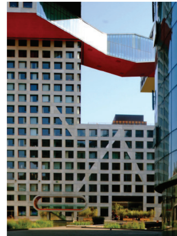
Figura 28: Fachada interna del edificio Linked Hybrid. Fuente: Obtenida de https://larryspeck.com/wp-content/uploads/2019/04/Larry-Speck-UTSOA-Stephen-Holl-Linked-Hybrid-Beijing-Housing-17-uai-720x900.jpg
