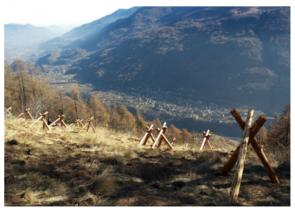
Fig. C21.5. Larch crib wall (left) and tripods (right) (Photos: CFAVS).
