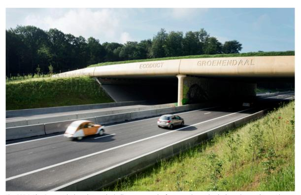
Fig. C28.6. The Groenendaal ecoduct ecologically reconnects the forest, cut in two by the busy ring road around Brussels (Photo: SVD Absoluut).
