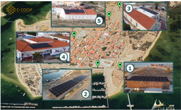
Figura 2. As 5 UPACs instaladas na aldeia da Culatra
